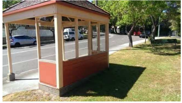
BS026: Southern and western elevations
