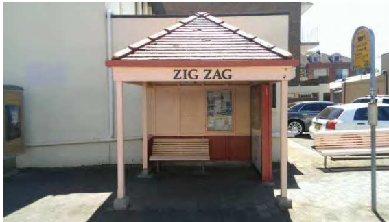
BS056: Looking north
