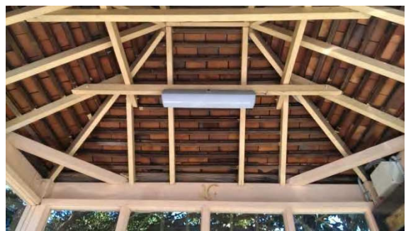
BS046: Interior roof
