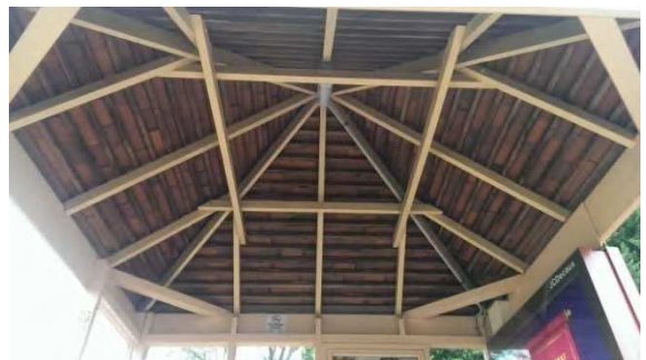
BS016: Internal roof
