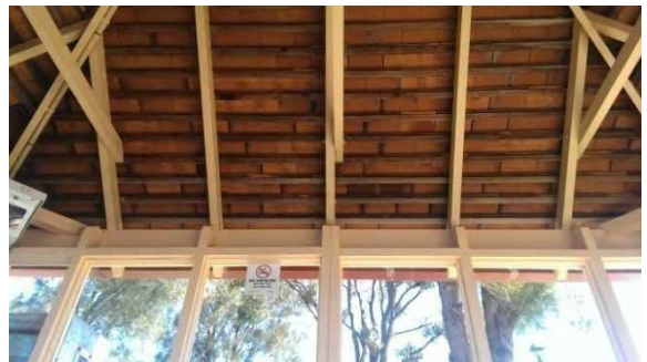
BS058: Interior roof
