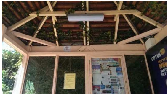
BS030: Interior roof
