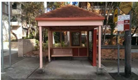
BS066: Front elevation looking south
