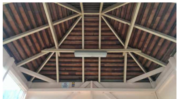
BS052: Internal roof
