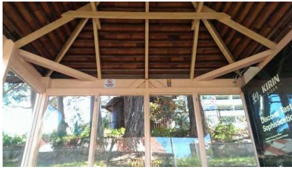
BS024: Interior roof
