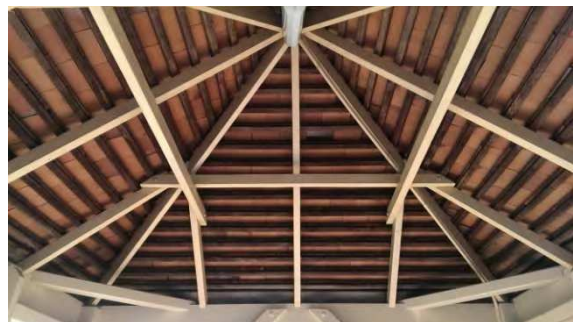
BS051: Internal Roof
