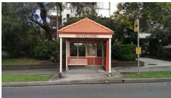
BS067: Front elevation looking south
