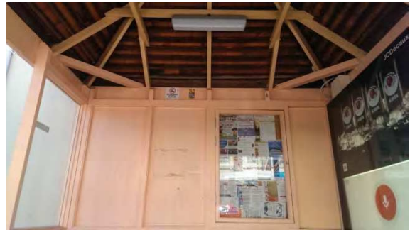
BS056: Interior Back and Roof
