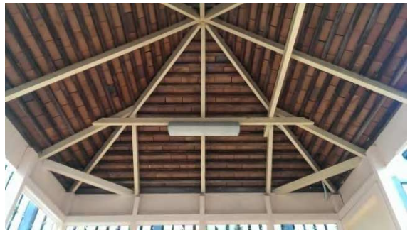
BS018: Internal roof
