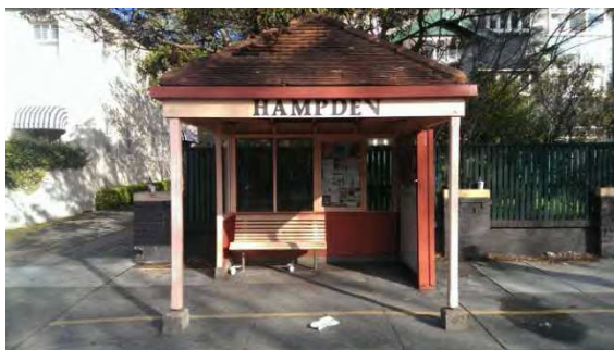
BS009: Front elevation, looking south
