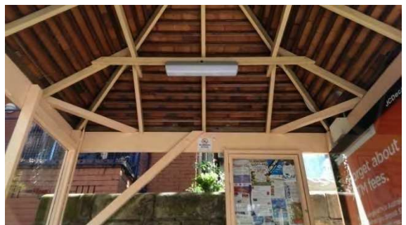
BS006: Internal roof
