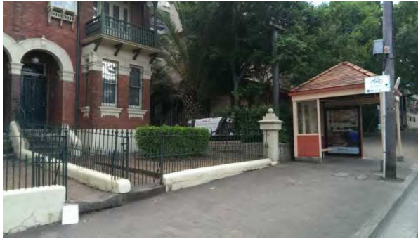
BS045: Adjacent buildings, looking north
