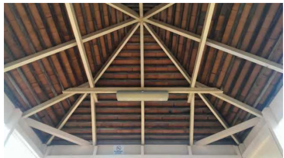
BS019: Internal roof
