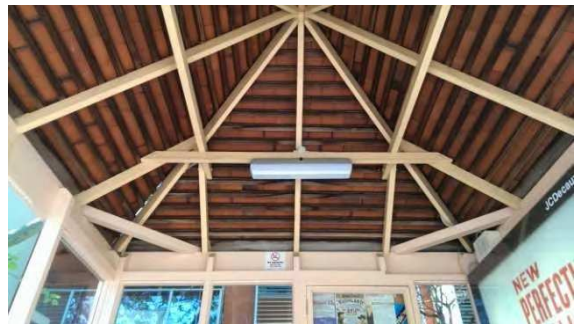
BS003: Internal Roof
