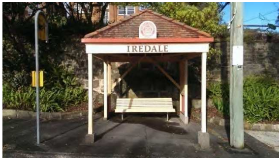
BS051: Front elevation, looking east
