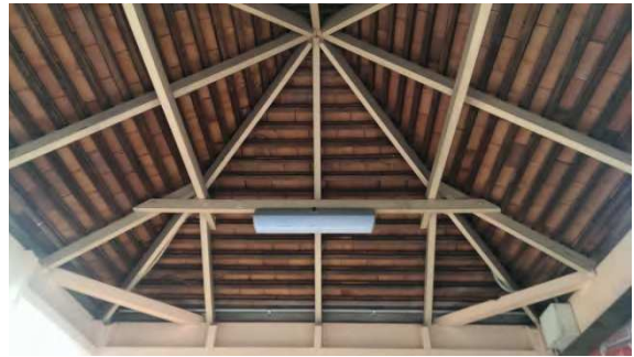
BS009: Internal Roof
