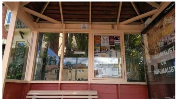
BS045: Internal roof
