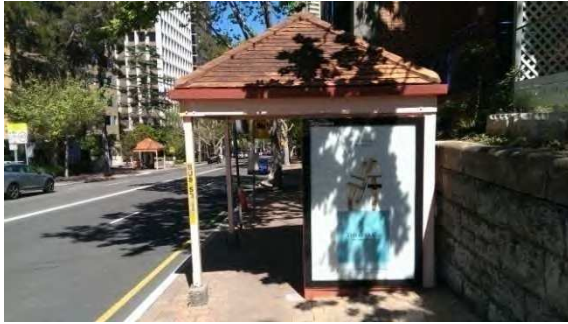
BS006: Northern elevation, showing advertising panel
