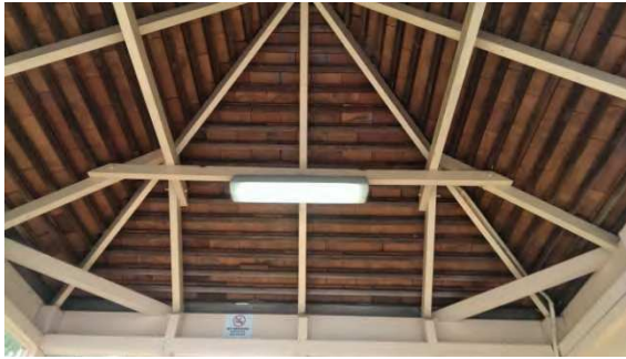
BS013: Internal roof
