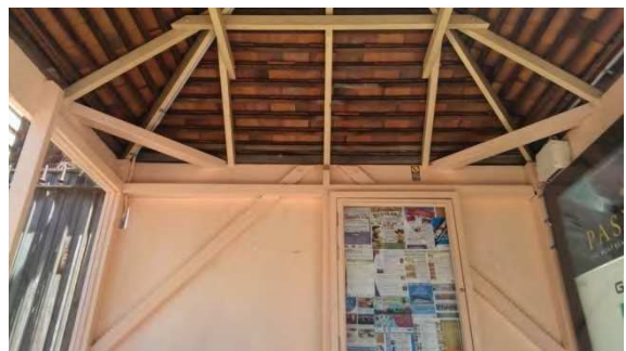
BS033: Interior roof
