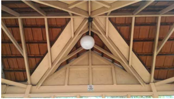
BS054: Interior roof and light
