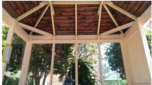
BS060: Interior back and roof
