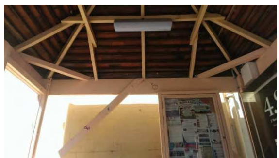
BS028: Interior roof
