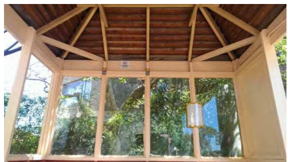
BS022: Interior roof
