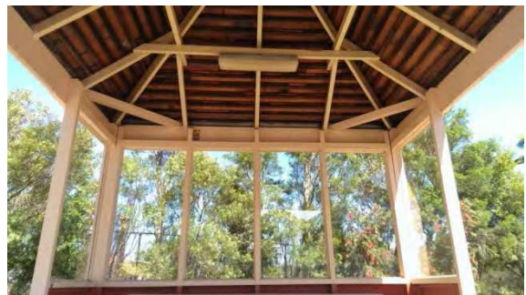
BS026: Interior Roof
