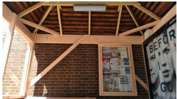
BS057: Roof and back wall
