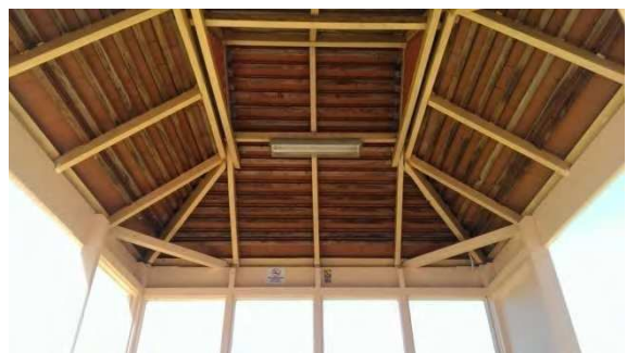
BS061: Internal roof
