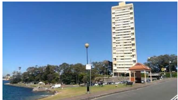
BS061: Street view, showing Blues Point Tower
