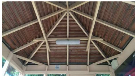
BS067: Internal roof
