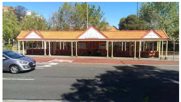
BS054: Front elevation, facing south
