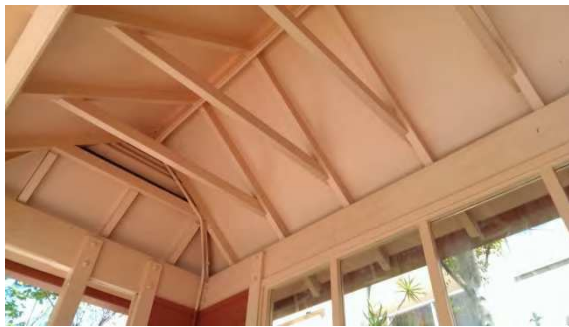
BS034: Interior roof
