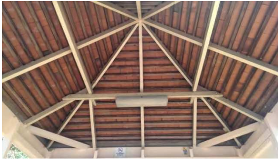
BS044: Interior roof
