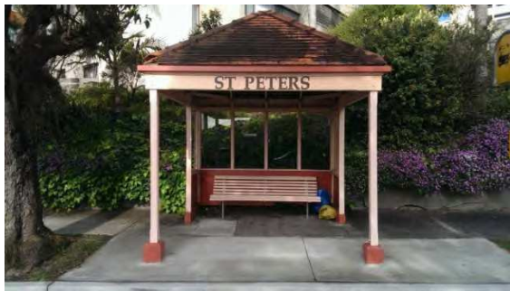
BS013: Front elevation, looking east
