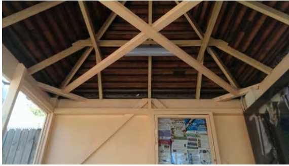
BS007: Internal roof
