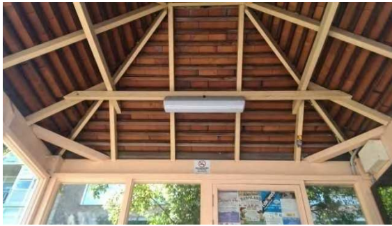
BS055: Interior roof
