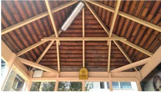
BS005: Internal ceiling
