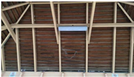
BS001: Interior of roof
