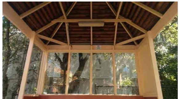
BS029: Interior roof
