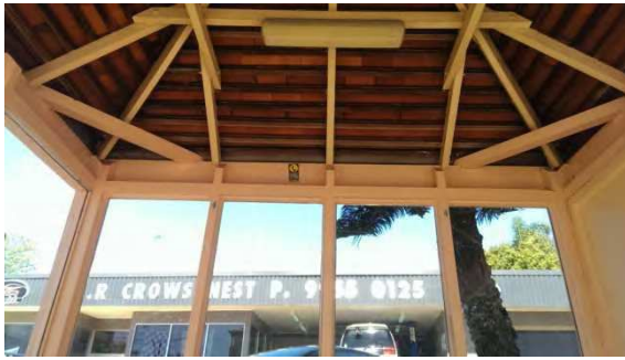
BS020: Interior roof
