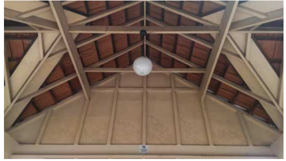
BS053: Interior roof
