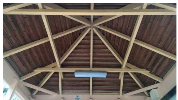
BS066: Internal roof
