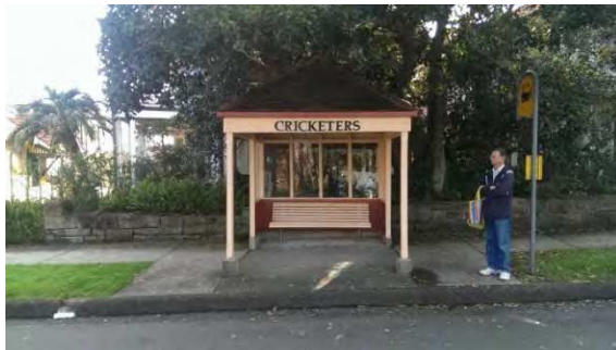
BS012: Front elevation, looking west
