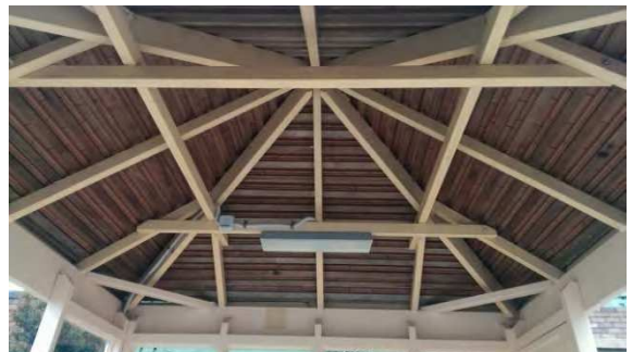
BS065: Internal Roof
