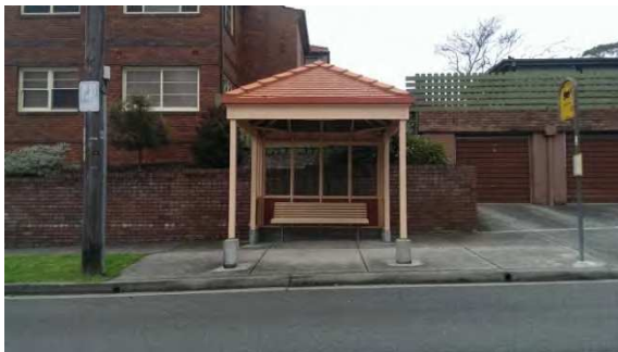
BS065: Front elevation looking west
