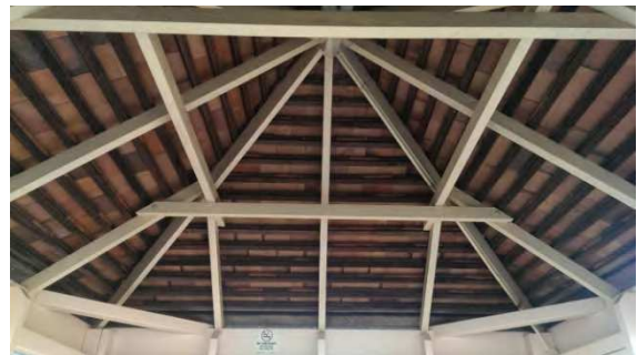
BS011: Internal Roof
