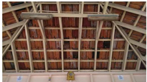
BS004: Internal ceiling
