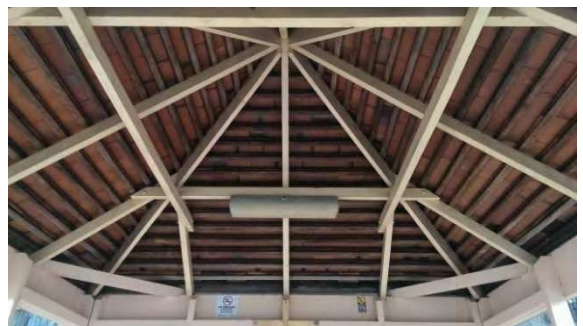
BS002: Internal Roof
