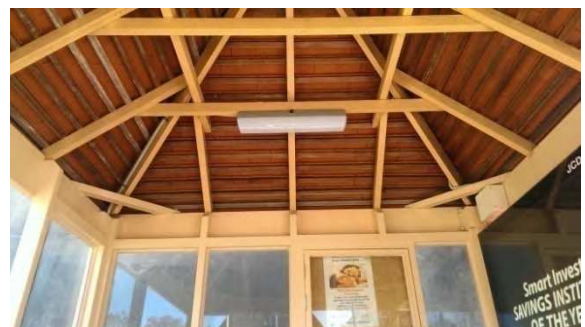
BS038: Interior roof
