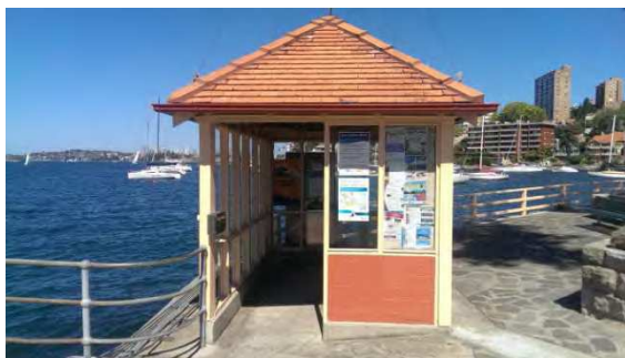
BS058: Eastern elevation, looking west
