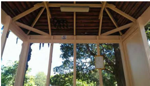
BS023: Interior Roof
