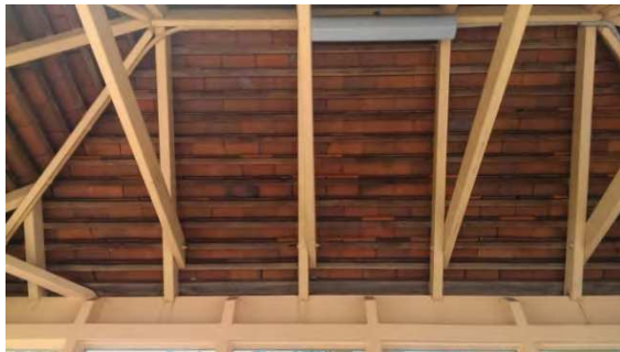
BS010: Internal Roof
