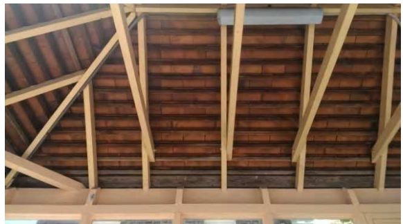
BS031: Interior roof
