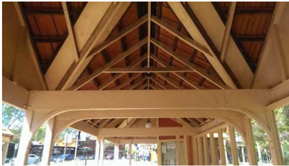
BS053: Interior roof
