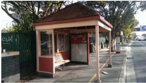
BS009: Looking west along Military Road
