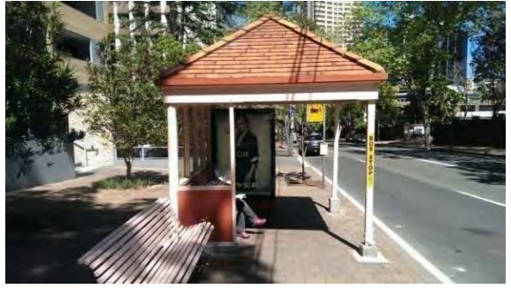
BS005: Northern elevation, with additional seat
