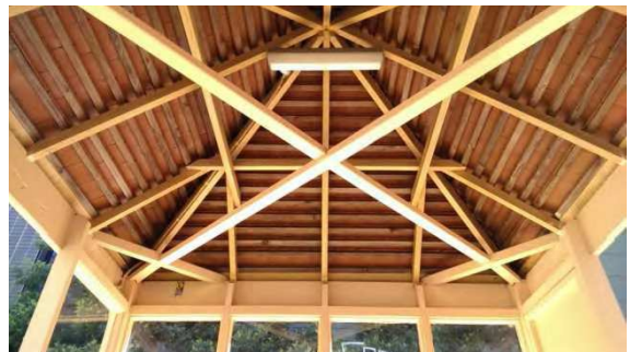
BS059: Interior roof
