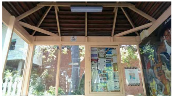
BS035: Interior back and roof
