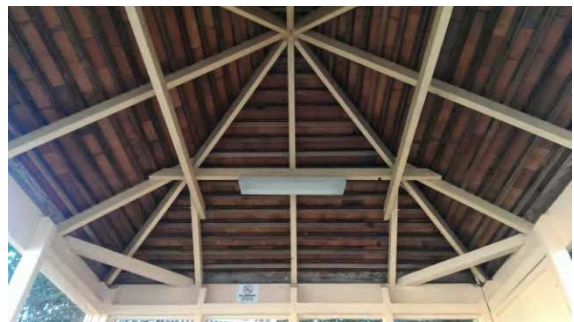
BS012: Internal Roof
