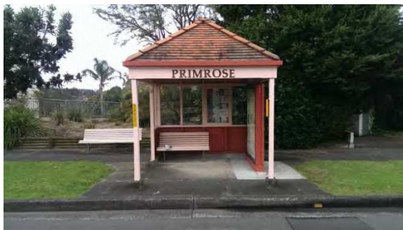
BS016: Front elevation, looking north
