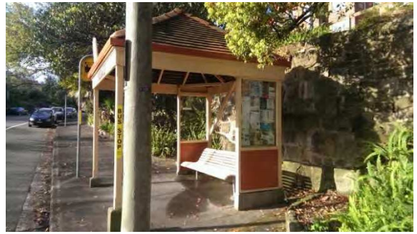
BS051: South elevation with community board
