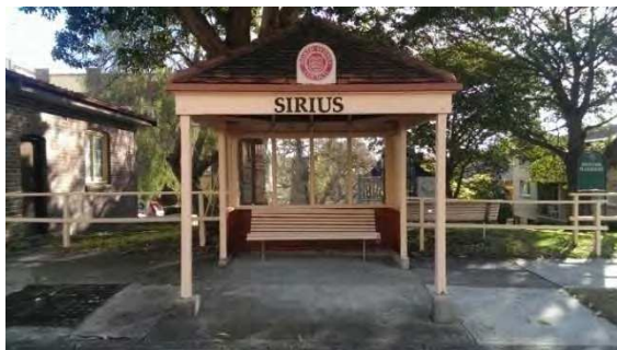
BS011: Front elevation, looking west
