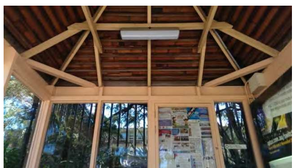
BS008: Internal roof
