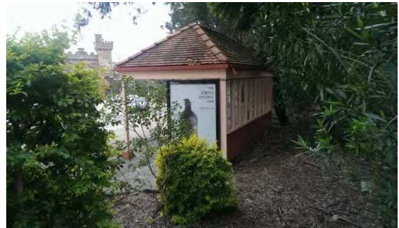
BS001: Southern/western elevations
